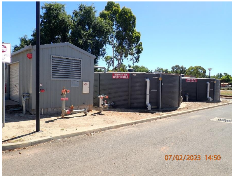
Photograph 04: View of the existing fire hydrant / sprinkler storage tanks
